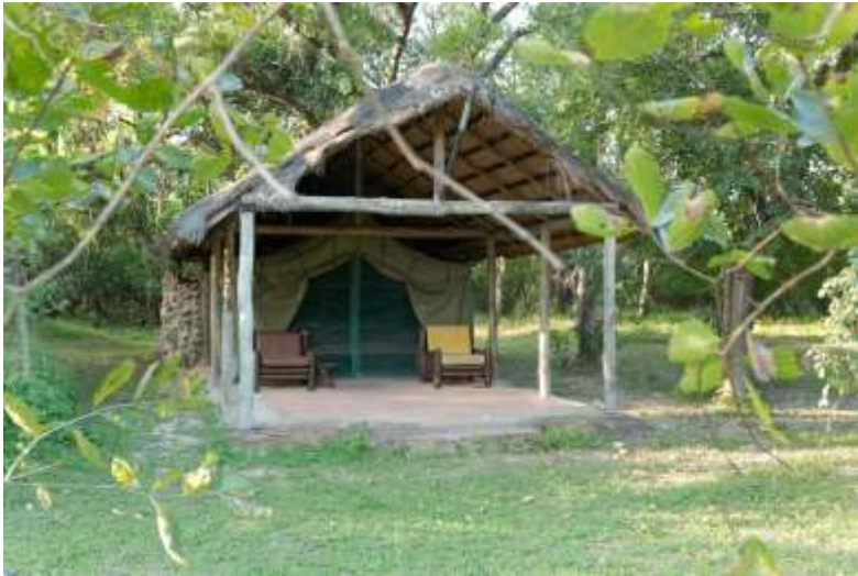
Figure 37. Example of a self-contained permanent tent from Hippo lodge, Mulola, Kafue park
